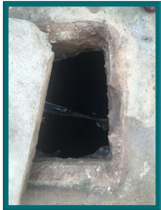
PLACENTA DISPOSAL UNIT IN THE CONCRETE FLOOR AT THE BACK OF THE MS UGANDA CLINIC, MATUGA
